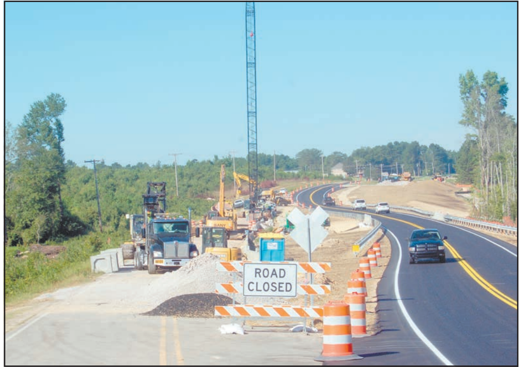
THE ROAD TO PROGRESS. Crews repaired a section of U.S. 401 that washed out following a storm. Improvements to U.S. 401 are underway, essentially from the Wake County line up to Royal. Plans to widen the two-lane highway all the way into Louisburg are still in the works, but have been delayed by available funding.
